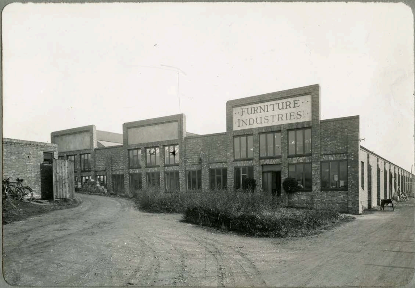
SOUTH WEST VIEW OF WORKS
